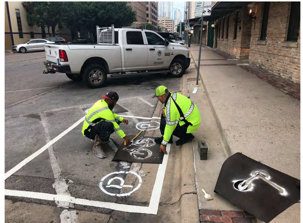
Image Source: City of Austin Transportation Department
